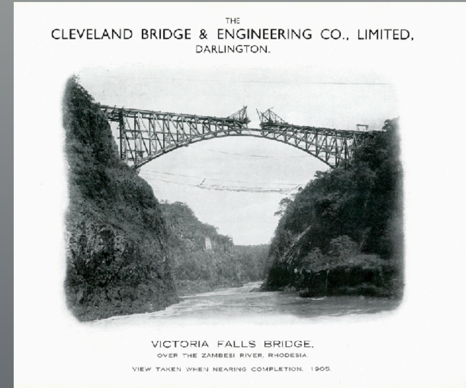
Victoria Falls bridge 1905
